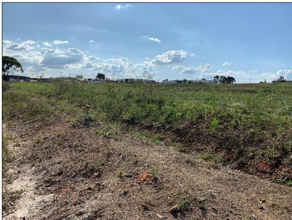
Photograph E4 – Existing drainage line on the southern boundary of the study area looking west.
