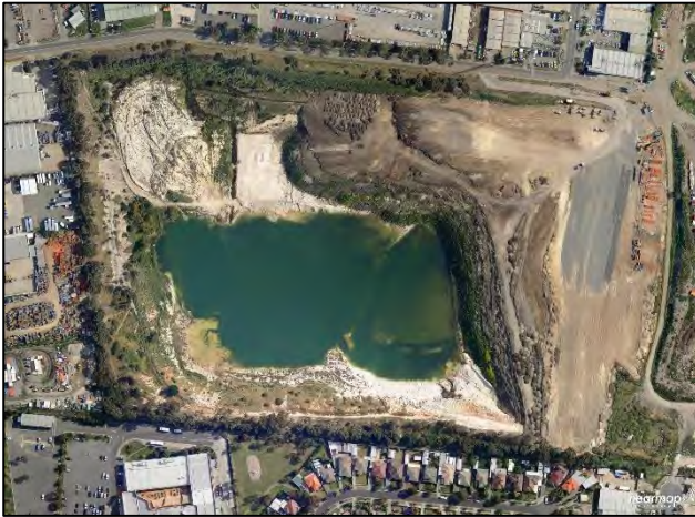
Plate 3. Progressive filling activities within the study area (Nearmap 23/10/2012)
