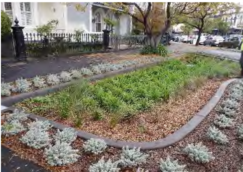
Figure 11 - Example of a streetscape bioretention system
