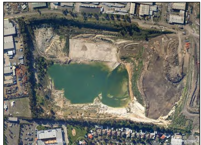
Plate 2. Progressive filling activities within the study area (Nearmap 20/08/2011)
